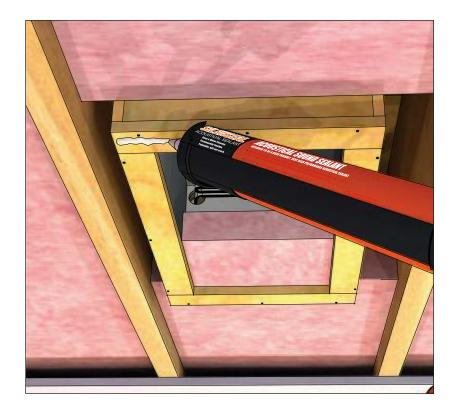
Apply a heavy dose of SilenSeal Acoustical Sealant to the bottom of the Backer Box flange before installing drywall.
