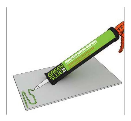
Cut 1/4" or 3/8" cement board to line the inside of the OSB box. Apply Green Glue to the back side of Cement Board and then apply.
