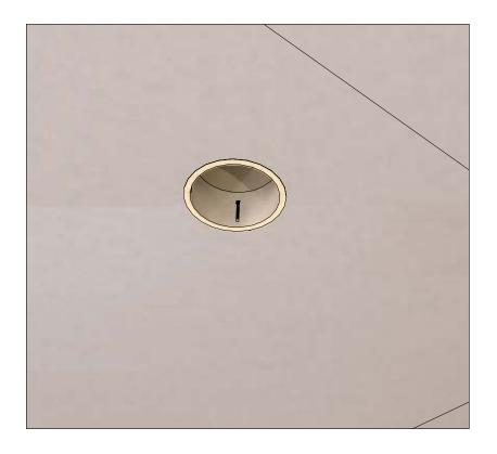
Hold light fixture against ceiling and push clips through the drywall hole.
