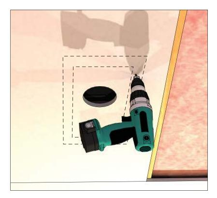
Secure the Backer Box flange with drywall screws. This will securely seal the Backer Box and SilenSeal Acoustical Sealant to the ceiling drywall.
