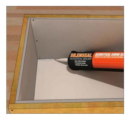
Seal the Cement Board edges with SilenSeal Acoustical Sealant.
