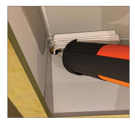
Seal the hole where the wire enters the box with SilenSeal Acoustical Sealant.
