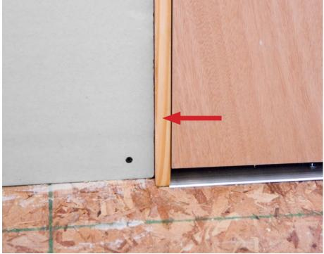
Ideally you would like to run drywall to the edge of door jamb and seal any gap with Acoustical Sealant.
