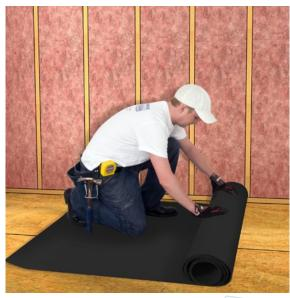
Place the roll of Mass Loaded Vinyl on the floor, then cut to length.
