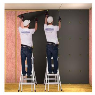
With the assistance of another person, position the first length of MLV in the top corner of wall. Ensure that the Mass Loaded Vinyl is straight along the ceiling so as to evenly drape the wall. Maintain an even gap along both the floor and ceiling.
