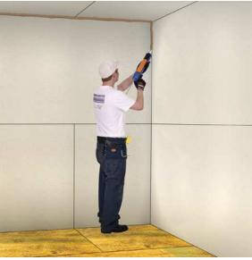
Hang your drywall over the MLV, vertically or horizontally. Caulk the perimeter seams with Acoustical Sealant. Proper sealing is necessary to achieve quality sound isolation results.
