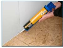
Apply SilenSeal Acoustical Caulk to any perimeter gap. Tape and mud as normal to finish the wall.
