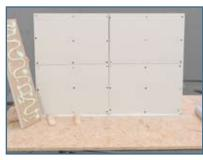
Apply Green Glue to back of the second layer of drywall, and hang it vertically. Press firmly to squeeze the Green Glue, then screw into place.
