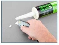
Use a utility knife and cut a 3/8" opening in the nozzle. A fat Green Glue bead is preferred.
