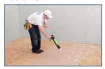
Apply the first tube of Green Glue in a random pattern. Make sure the floor is clean so not to damage the face of the drywall. You may also consider using sawhorses and set drywall on.
