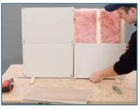
Screwing the drywall in place, following local building code. Note the optional spacer on the floor. Fill with SilenSeal Acoustical Caulk before applying second layer.
