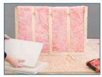
Staggering drywall seams between layers is important for best performance. Here we're hanging the first layer of drywall horizontally on the sample model.
