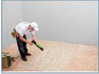
Apply the second tube filling in any large empty areas. The important thing is to apply the Green Glue approximately evenly over the board. There is no optimal pattern.
