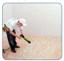
Apply 1-2 tubes of Green Glue in a random pattern to the backside of the second layer of drywall.
