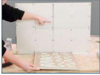
The next board will cover the seam of the first layer of drywall. All screws for all layers are installed into the studs or joists following local building code.
