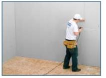
Screw the second layer of drywall to framing, following local building codes. (Use screws not nails)
