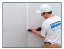
For best performance use SilenSeal Acoustical Sealant to seal any gap. You do not have to mud and tape the first layer of drywall.
