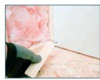
If you decide to leave a gap, place ¼" shims on the floor. Later you will fill in with flexible caulk. Alternately, you can install the drywall directly on the floor.
