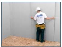
Press drywall into place. Make sure you stagger the seams of your drywall layers. You do not want your seams from layer 1 to align with the seams of layer 2.
