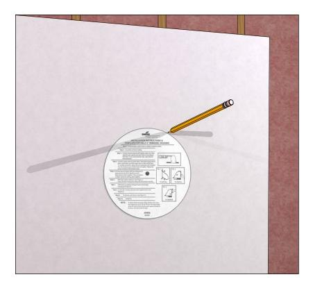
When you are ready to install the ceiling drywall, pre-mark the holes for the ceiling-can. Use the manufactures template to acquire a tight fit. Double check with a dry fit and then cut the hole before installing the drywall.
