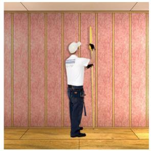
Measure the distance between the floor and the ceiling. Subtract 1/8" - 1/4" from the measured length.
