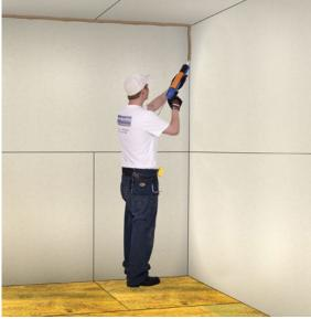
Hang your drywall over the MLV, vertically or horizontally. Caulk the perimeter seams with Acoustical Sealant. Proper sealing is necessary to achieve quality sound isolation results.
