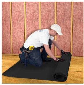
2 Place the roll of Mass Loaded Vinyl on the floor, then cut to length.
