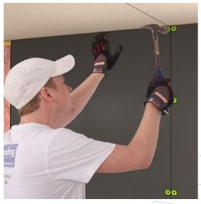
For 16" On Center (O.C.) framing, hammer the nail and washer through the MLV every 24" o.c. along the top plate length of each stud.
