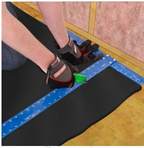
3 Use a T-Square or Straight Edge to cut a square edge. Use a Utility Knife and cut the MLV to length.
