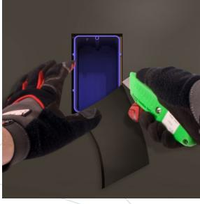
Be careful not to cover electrical outlets boxes. It is best to expose the outlets boxes as you install each length of MLV.
