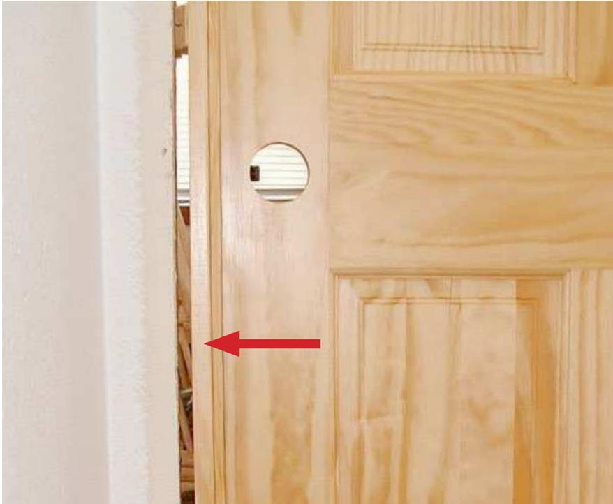
Typically a large gap between the drywall and the door jamb is left when a door is installed. This is a great spot for sound to leak through.
