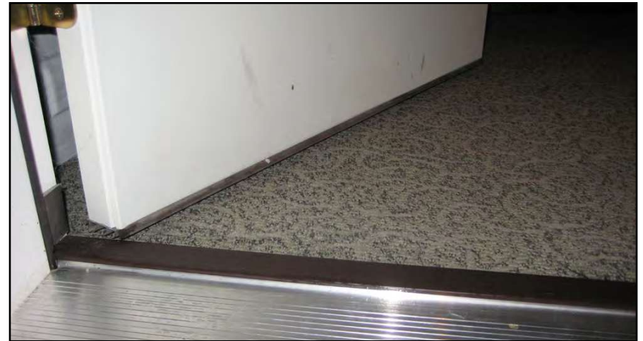
Metal door threshold that accompanies a standard exterior door.
